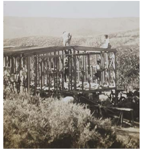
Skyline Lodge under construction in the summer of 1946 – 47 which became the first ski lodge in Falls Creek. In 1946, Toni and Skippy St Elmo lived in a two room hut near the existing road beside the creek down the gully to be known as Falls Creek. Pic – Courtesy the St Elmo collection.
